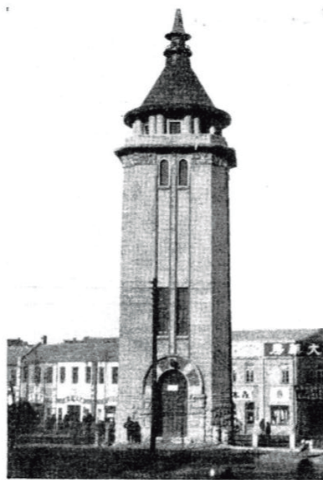
Transport Station of Electricity
